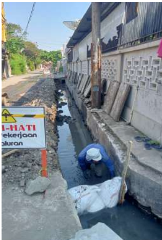
Gambar 4.8 Galian Crossing Drainase Eksisting (Sumber : CV. Progresif Quality Planning, 2023)
