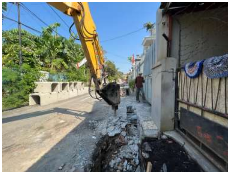
Gambar 4.7 Galian Drainase Eksisting (Sumber : CV. Progresif Quality Planning, 2023)
