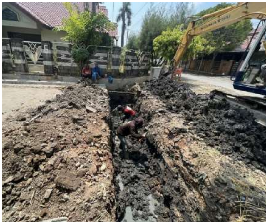
Gambar 4.11 Galian Crossing Pekerjaan Box Culvert (Sumber : CV. Progresif Quality Planning, 2023)
