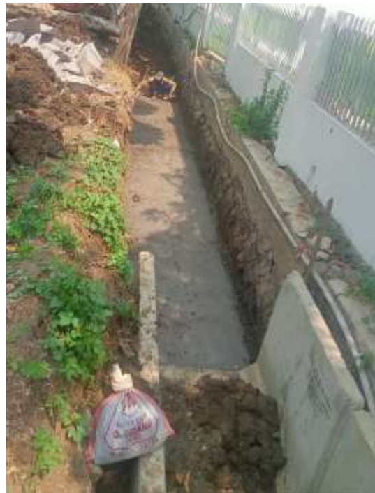
Gambar 4.9 Lantai Kerja U-Ditch (Sumber : CV. Progresif Quality Planning, 2023)
