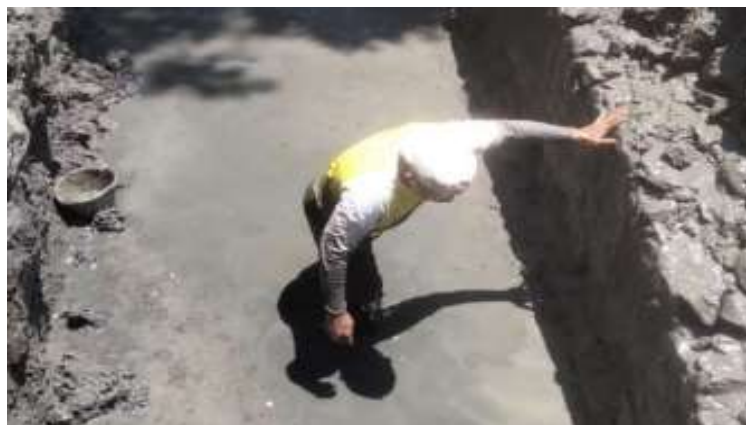
Gambar 4.12 Pengecoran Lantai Kerja Box Culvert (Sumber : CV. Progresif Quality Planning, 2023)
