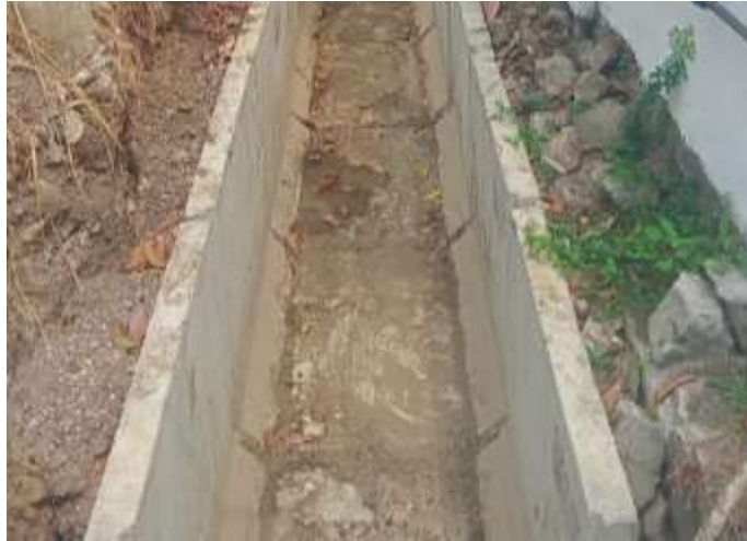
Gambar 4.10 Penyambungan U-Ditch (Sumber: CV. Progresif Quality Planning,2023)
