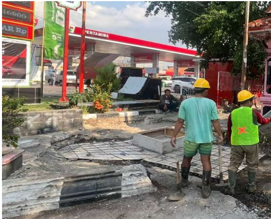
Gambar 4.14 Pembesian Manhole (Sumber : CV. Progresif Quality Planning,2023)
